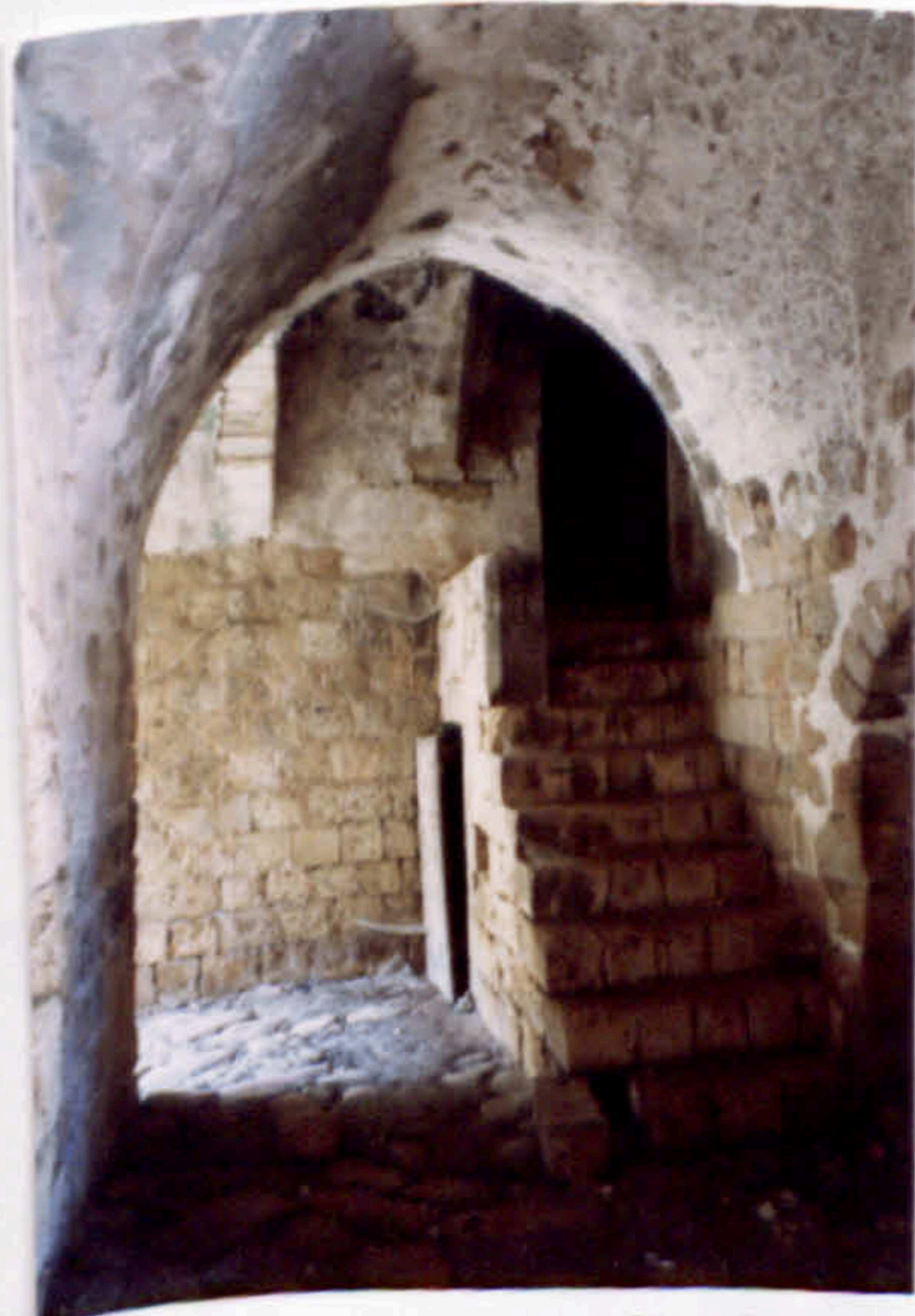
bent entry vestibule
