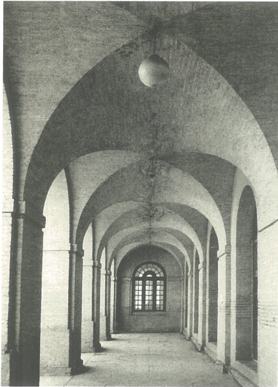
VIEW OF THE VAULTED GALLERY
