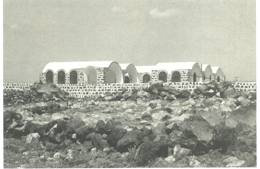
VIEW OF THE SCHOOL IN CONTEXT
