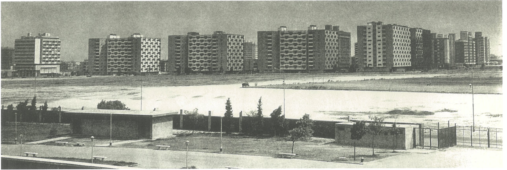
GENERAL VIEW OF THE APARTMENT BUILDINGS
