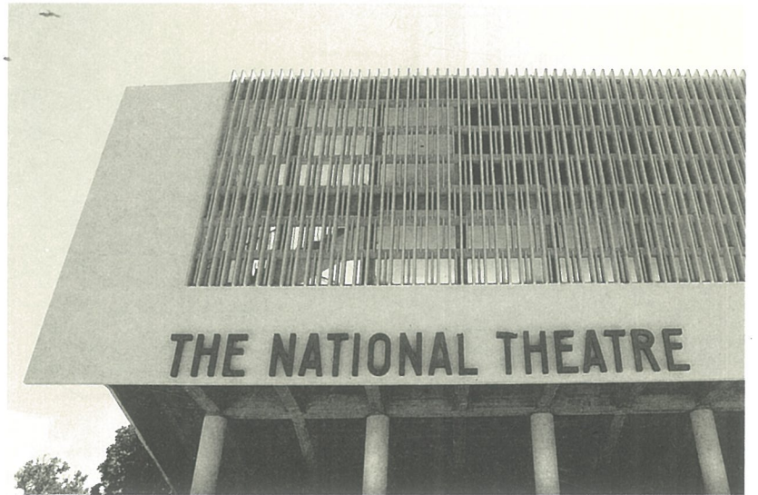
DETAIL OF THE MAIN ELEVATION
