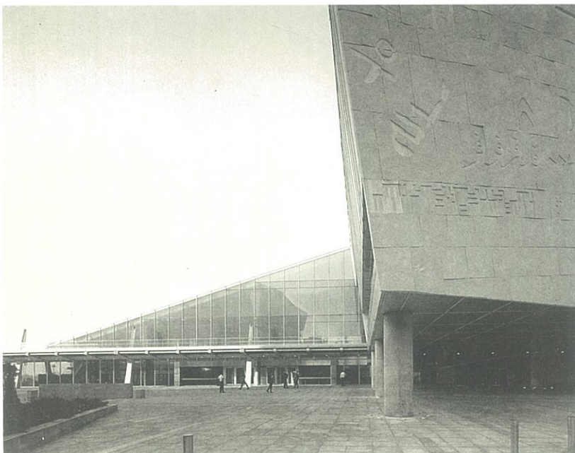
VIEW TO ENTRANCE
