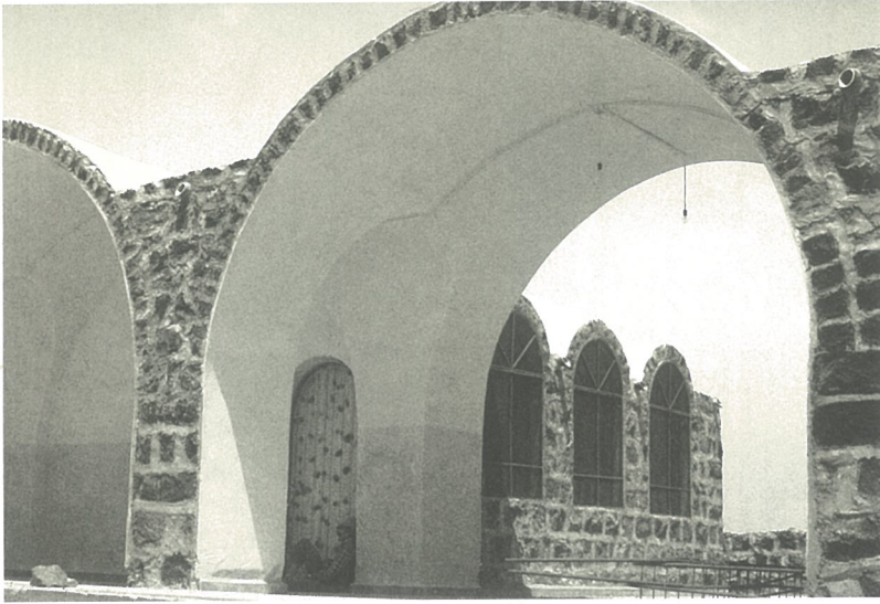
DETAIL OF BASALT VAULT
