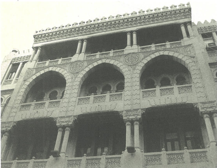
DETAIL OF THE MAIN ELEVATION
